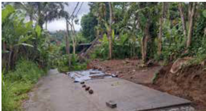
Membantu Pengembangan Pelebaran Jalan di Ubud Support for the Expansion of Road Infrastructure in Ubud
